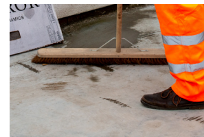
Clean the area
