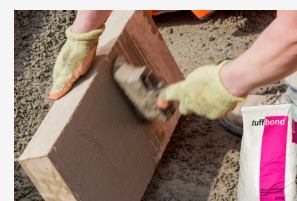
Apply tuffbond to concrete base and paving unit
