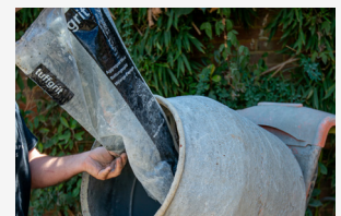
Mix binder and aggregate 1 binder : 4 aggregate
