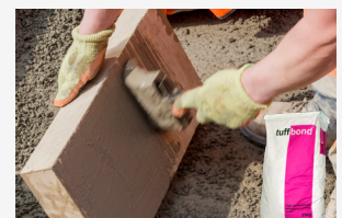
Apply tuffbond to concrete base and paving unit
