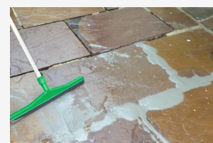
Spread mortar to fill joints and remove excess
