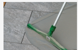
Spread tuffjoint Utility to fill the joints
