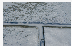
Spray water over the joints
