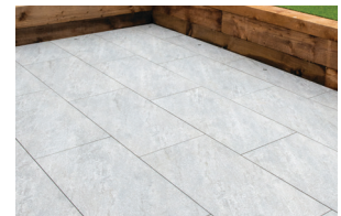
Clean the area
